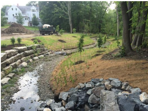
Figure 3-3. Example of a Stream Restoration Project with Floodplain Connection
