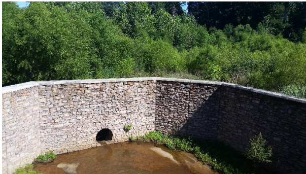
Figure 2-16. Example of a Functional and Well-Maintained Stormwater Management Structure
