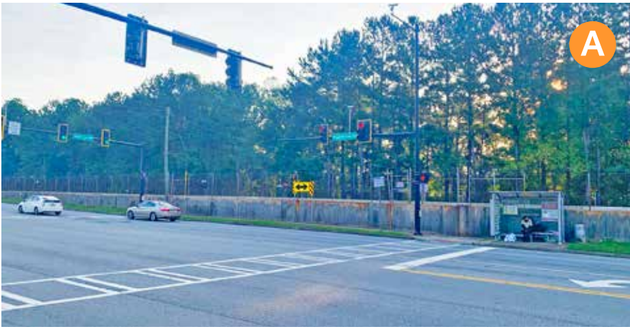
Existing MARTA bus stop conditions are located along the east side of Peachtree Road in the narrow space between the wall and traffic.
